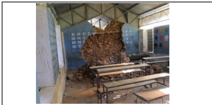
Figure 5. Earthquake damage at Shree Birendra Secondary School, Nuwakot Source: Room to Read
